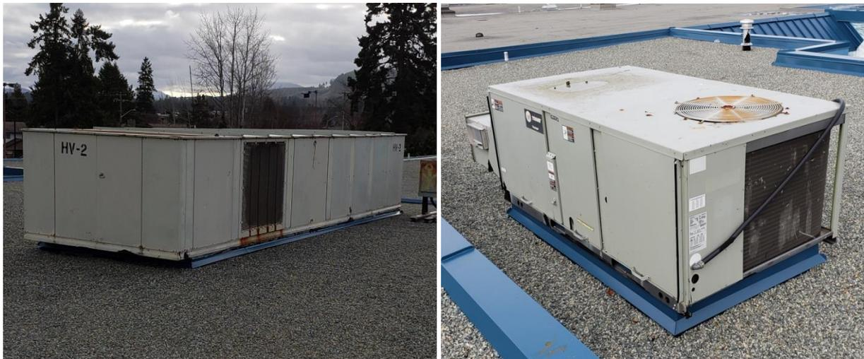
**Figure 27: HV2 and HV4 rooftop units with DX cooling**
