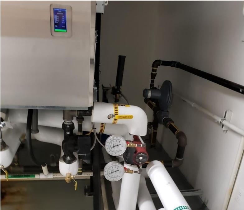
**Figure 2: B-1 supplies both DHW and space heating via two boiler pumps**
