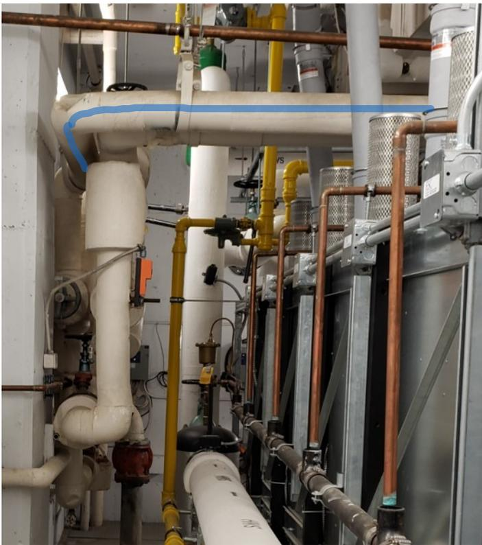
**Figure 28: Basement mechanical room. Chiller water pipe marked in blue. The boilers are on the right.**
