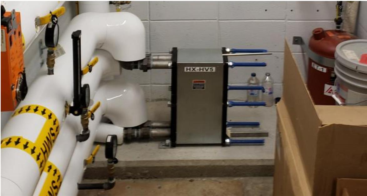
Figure 4: HX-HV5 heat exchanger
